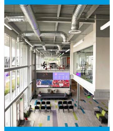
The smartengine deployment of "the link" in Nocatee, Florida has an incredible LPD of 0.12 watt/ft².
